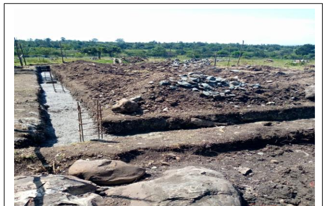
Working on footer & foundation Bomet
